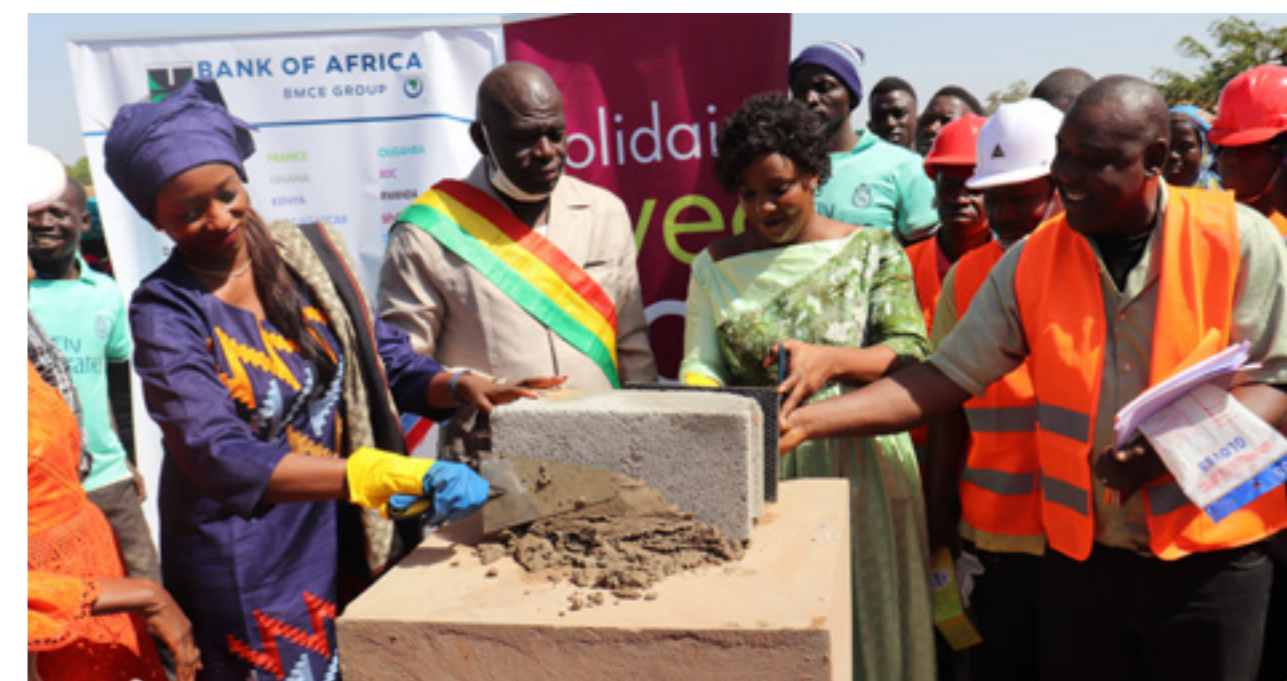
Laying of the first stone for the renovation of the basic school of Sirakoroni
